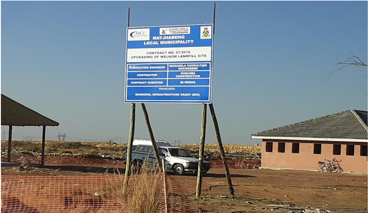
Figure 12: Welkom landfill under construction
