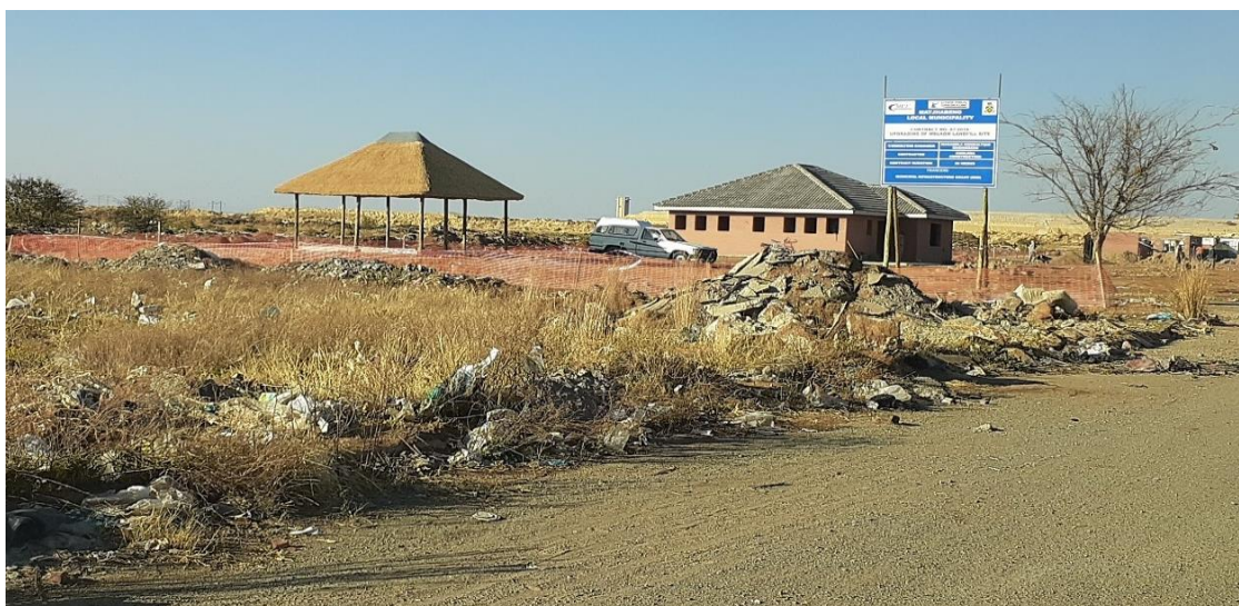
Figure 21 Welkom landfill site under construction (August 2019)
